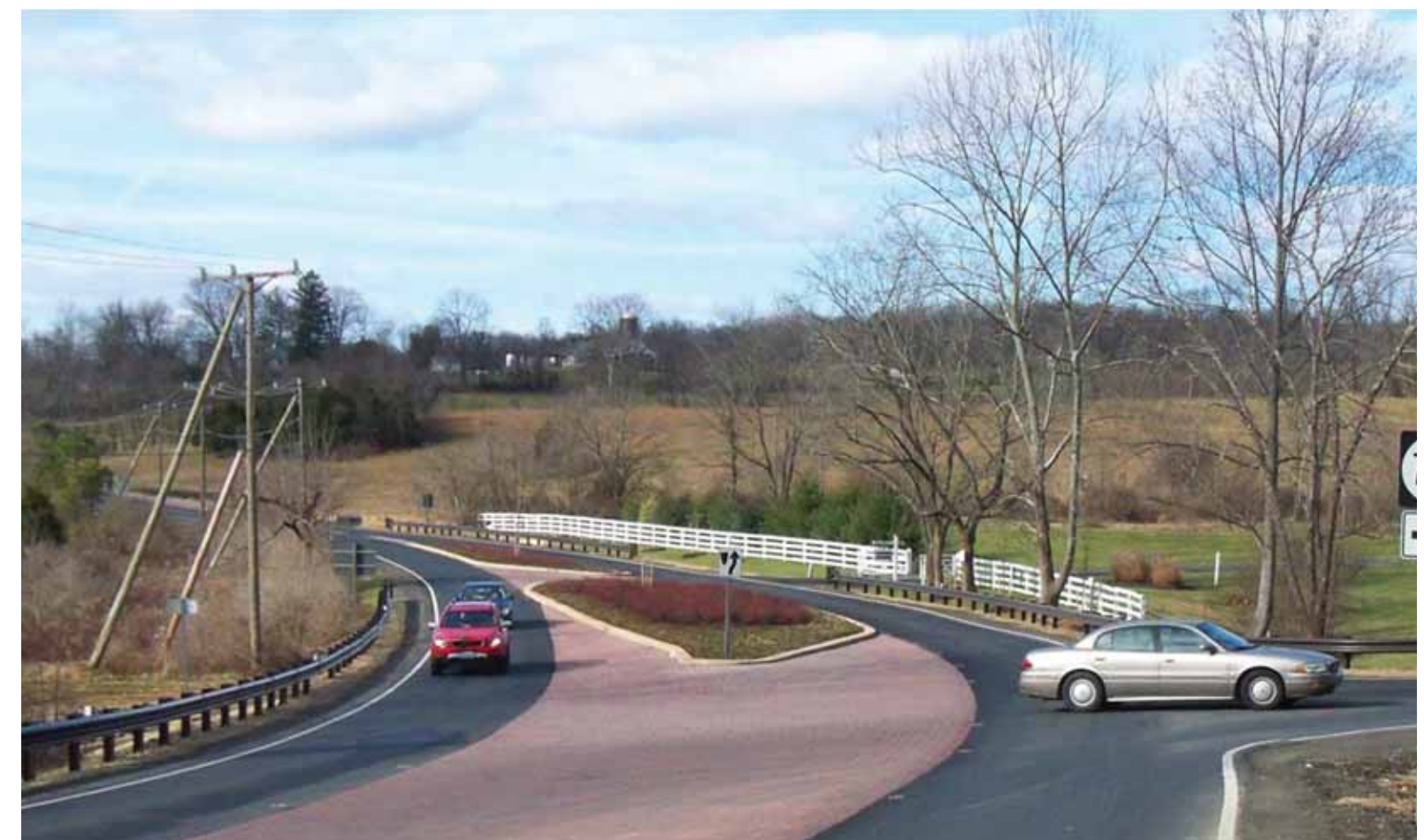
Splitter with pavers at intersection
