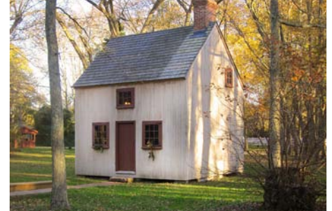
Figure 62 – Coxe Hall Cottage in Cold Spring Village
