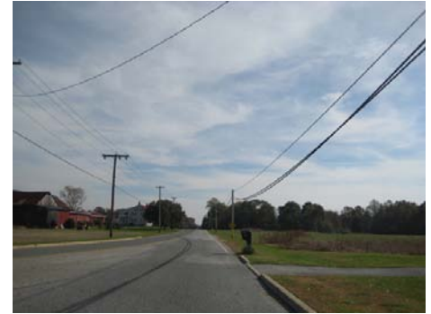
Figure 141 –Curb requirements may be waived by the appropriate municipal approving agency, and shoulders and/or drainage swales used when it can be shown that: shoulders are required by CAFRA; soil and/or topography make the use of shoulders and/or drainage swales preferable; and/or the community desires to preserve its rural character by using shoulders and/or drainage swales instead of curbs
