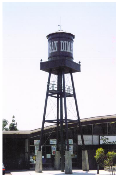
Figure 106 – Example of cell tower disguises as a water tower
