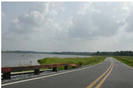
Figure 140 –Steel-backed wood guardrails are ideal for marine environments where corrosion is a problem
