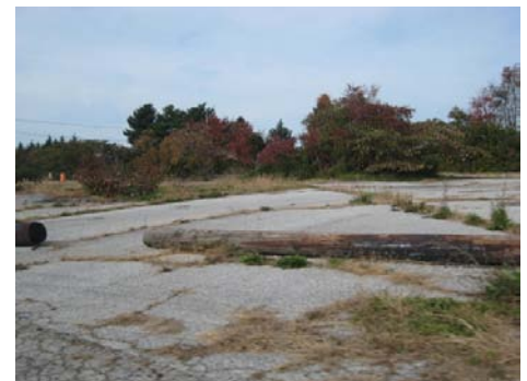
Figure 103 – Example of abandoned property in need of rehabilitation: remove asphalt and plant to grass until property is redeveloped
