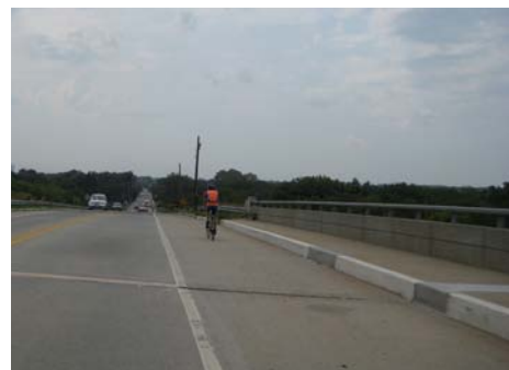
Figure 137 – A bridge with adequate space for bicycles and pedestrians
