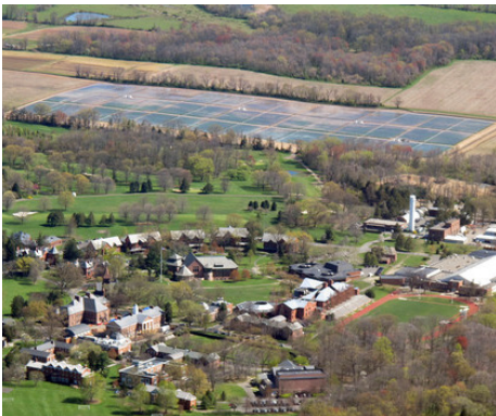
Figure 97 – Monitoring utility installations is an important issue for the Bayshore Heritage Byway. Solar installation at Lawrenceville School near Route 206 in central NJ illustrates the scale of some recent installations.
