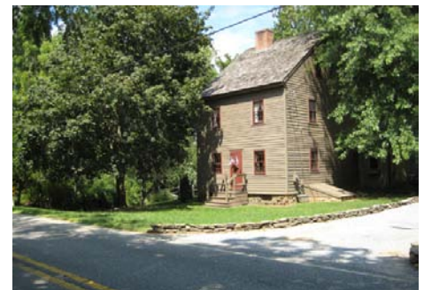
Figure 5 – Greenwich Historic Architecture
