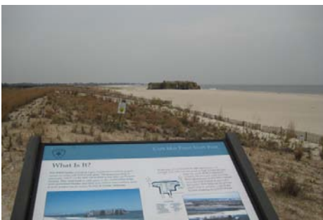
Figure 61 – Cape May Point State Park World War II Bunker
