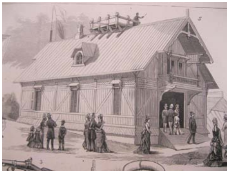
Figure 124 –1876 Life-Saving Station is being reconstructed along the Delaware Bay at Sunset Beach
