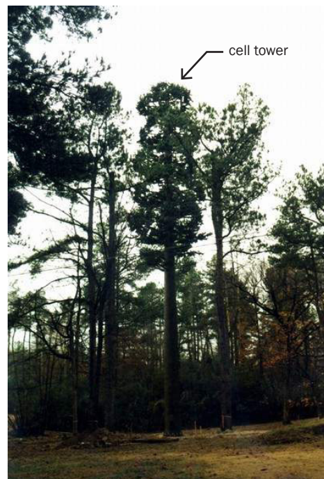
Figure 107 – Example of more appropriate use of camouflage to reduce visual contrast of a cellular communication tower
