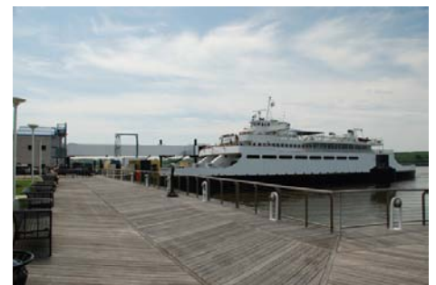
Figure 15 – Cape May – Lewes Ferry Terminal
